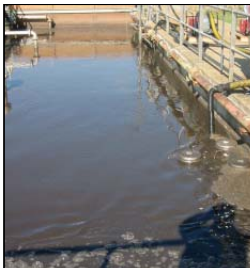
➤ Sewage tank after skimming cycle
